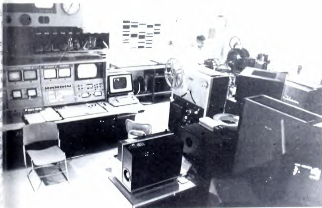
A view of the master control room at WLWD, Dayton, Ohio (an Avco station). Note the Vital Industries' automation system on the extreme right of the switching console.
